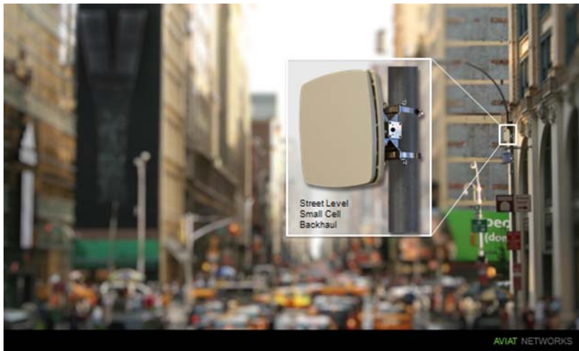
Figure 1 -- Sample Installation of Waivered Antenna
